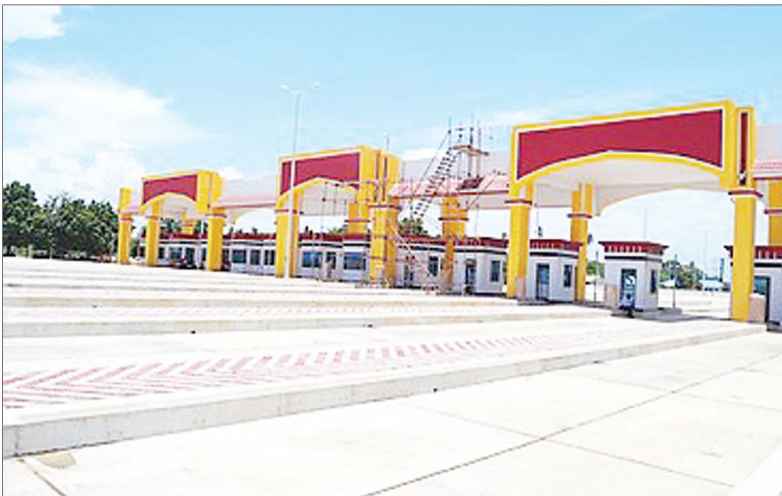
Nyerere Bridge toll booths
