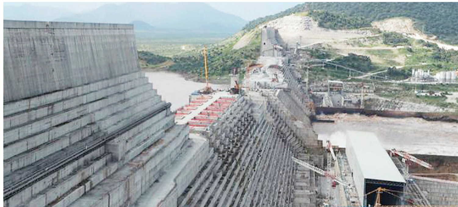
Ethiopia's Grand Renaissance Dam under construction on September 26, 2019.
