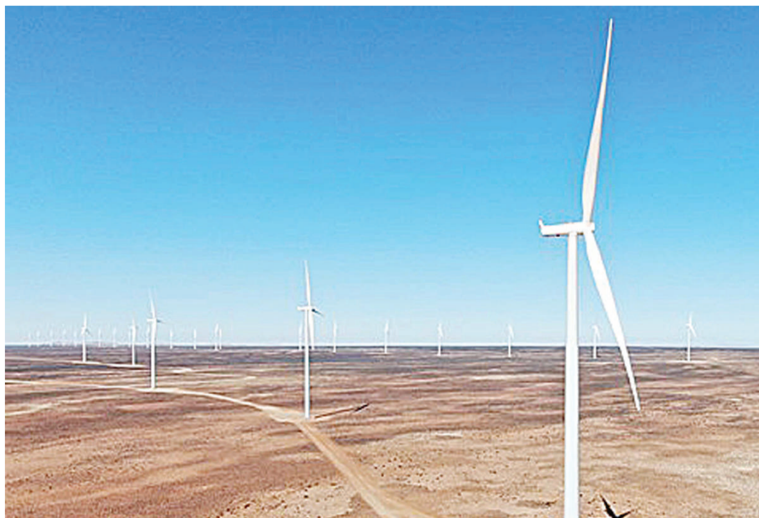
Kangnas Wind Farm of Springbok in South Africa's Northern Cape
