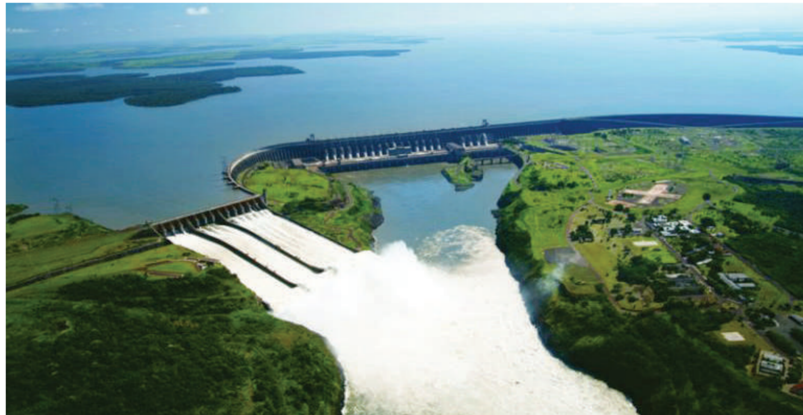
The Itaipu binational hydroelectric power plant, shared with Paraguay, was the last large, low-cost plant to be located close to major consumer markets. Inaugurated in 1984 on the Paraná River, on the border with Paraguay and close to Argentina, its installed capacity is 14,000 megawatts. Brazil's hydroelectric potential since then has been limited to rivers in the Amazon rainforest, with more expensive construction costs and the need for long transmission lines to large consumers. CREDIT: Itaipu Binacional
