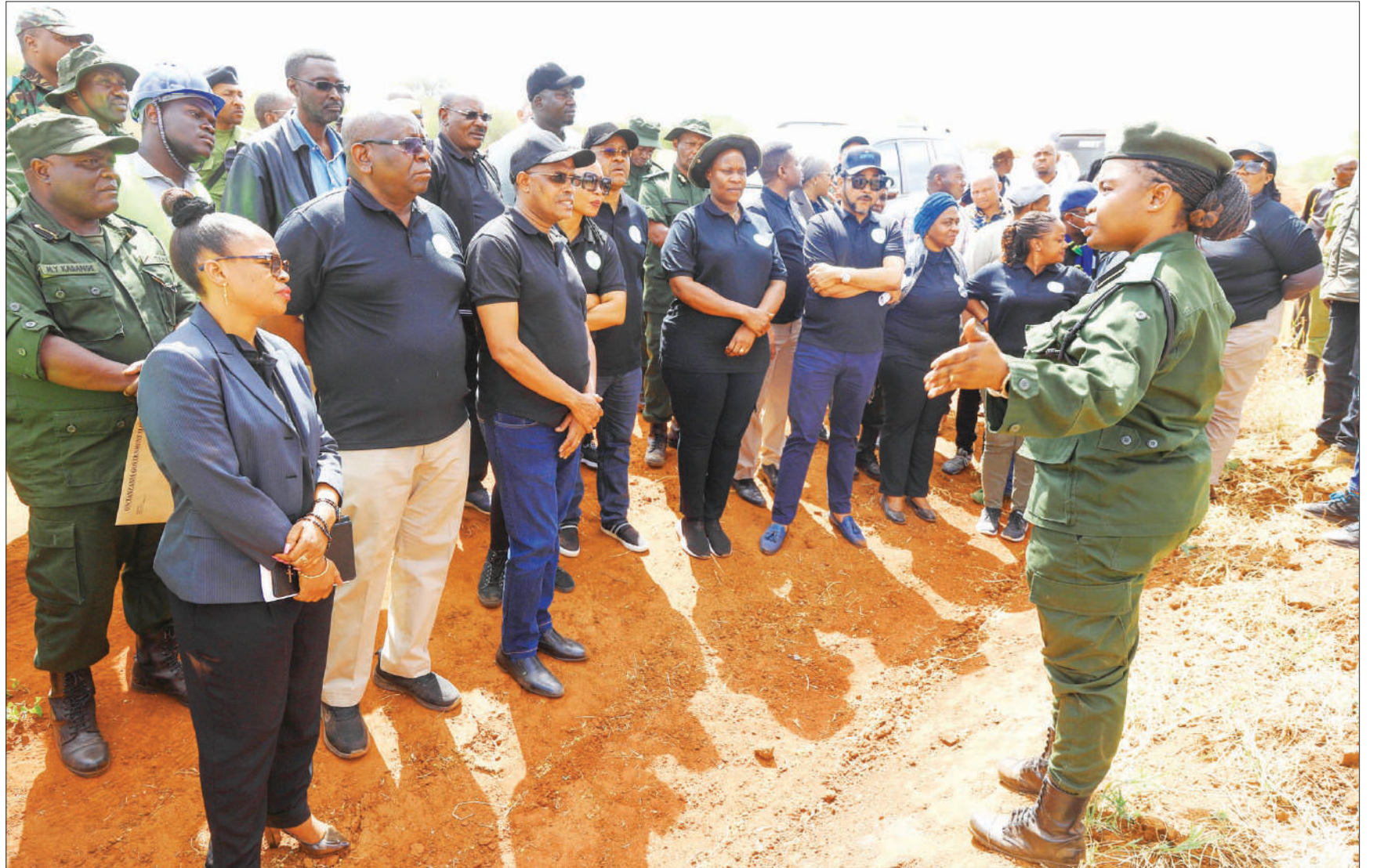
Tanzania Wildlife Management Authority deputy commissioner Khadija Malongo (R) pictured yesterday briefing members of the Parliamentary Standing Committee on Budget on the implementation of a 47.2-km road construction project in the Mkungunero Game Reserve in Kondoa District, Dodoma Region. Photo: Guardian Correspondent
