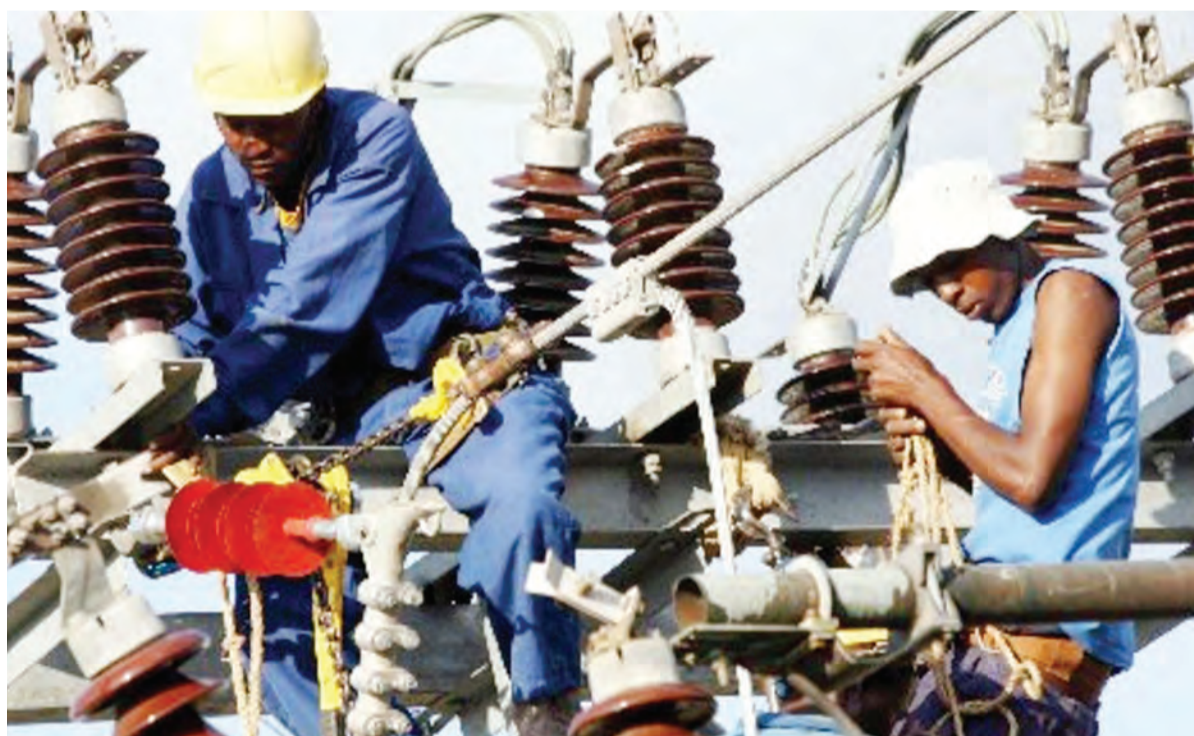
Kenya Power workers repair a power supply line.
