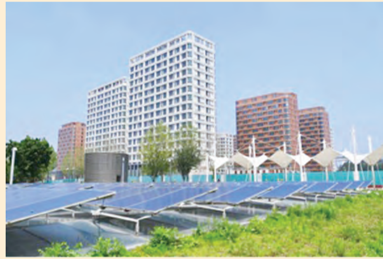
The Winter Olympic Village is completed and delivered to the Beijing Organising Committee for the 2022 Olympic and Paralympic Winter Games on June 26, 2021. The village, consisting of 20 residential buildings, covers an area of 330,000 square meters. It is divided into residential and operational sections. Photo shows the photovoltaic power generation system of the Winter Olympic Village. File photo
