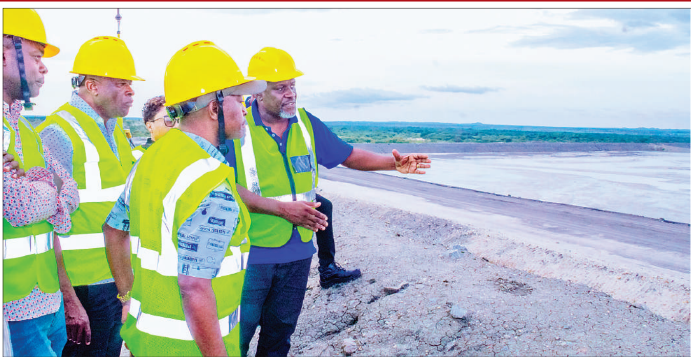
Shaghembe Mipawa (gesturing), chief engineer with Mwadui Diamond Mine in Shinyanga Region, pictured yesterday briefing visiting members of the Parliamentary Standing Committee on Energy and Minerals on the new mud storage dam currently being used in diamond production activities after the previous one collapsed, causing harm to local residents. Photo: Correspondent Marco Maduhu
