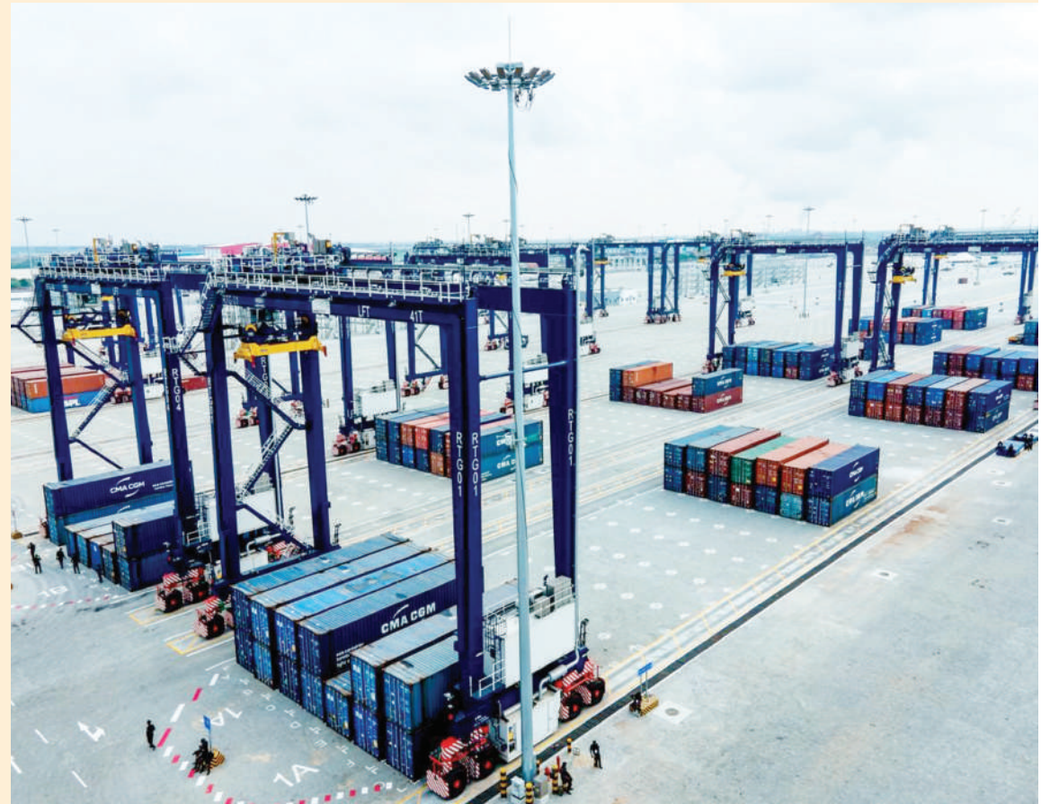
Photo shows the Lekki deep seaport in Nigeria. (Photo from the China Harbour Engineering Company Ltd.)
