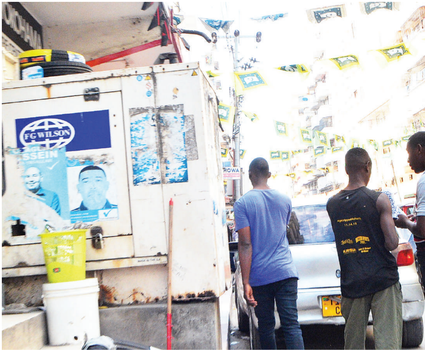
The standing of a heavy-duty generator in a pavement near the junction of Dar es Salaam's Livingstone and Mchikichi streets is making life difficult for pedestrians, as witnessed yesterday by Correspondent Miraji Msala
