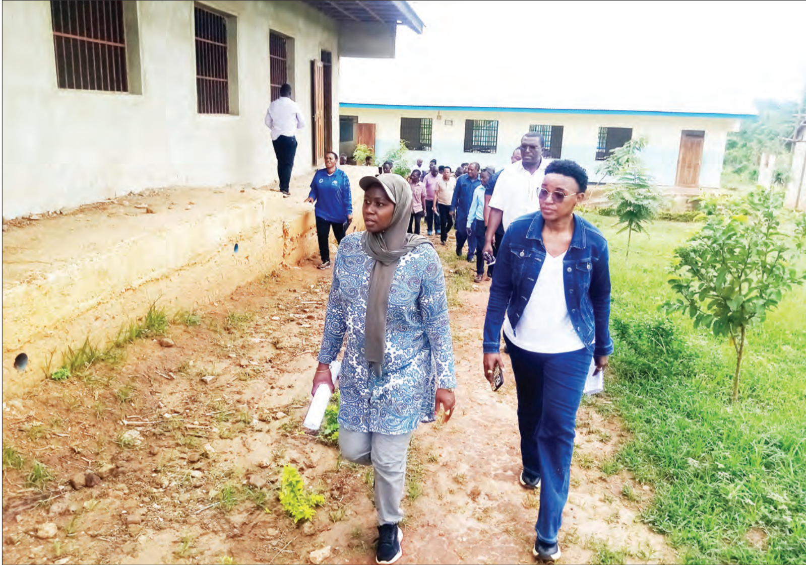
Parliamentary Local Government Accounts Committee chairperson Halima Mdee (R) pictured yesterday leading members of the committee in assessing progress in the construction of Chatuu Secondary School in Muheza District and, shortly later, Muheza District Hospital. Photo: Correspondent Steven William
