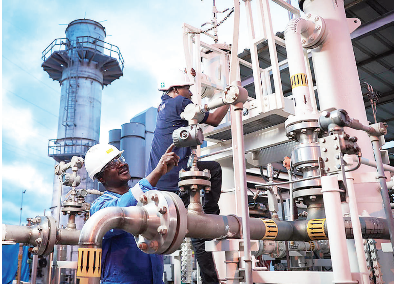
Songas Ltd's engineers at work.
