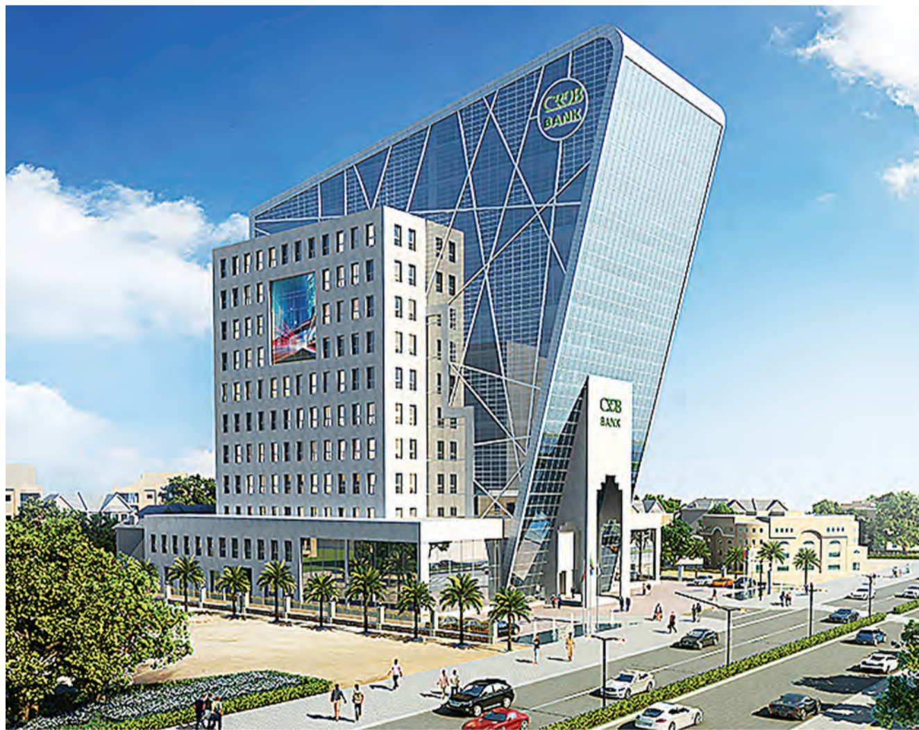
New CRDB Bank headquarters building under construction in Dar es Salaam.
