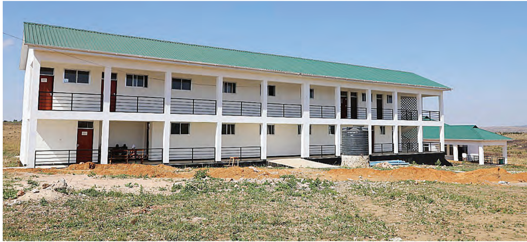
Buhigwe District Hospital building which is still under construction
