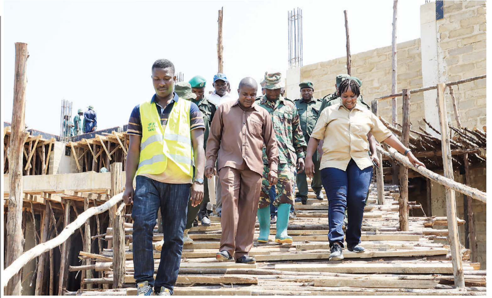
Natural Resources and Tourism deputy minister Mary Masanja (R) leaves a Tanzania National Parks three-star hotel building under construction at Chato in Geita Region recently in the company of, among other people, Chato district commissioner Charles Kabeho. Photo: Guardian Correspondent
