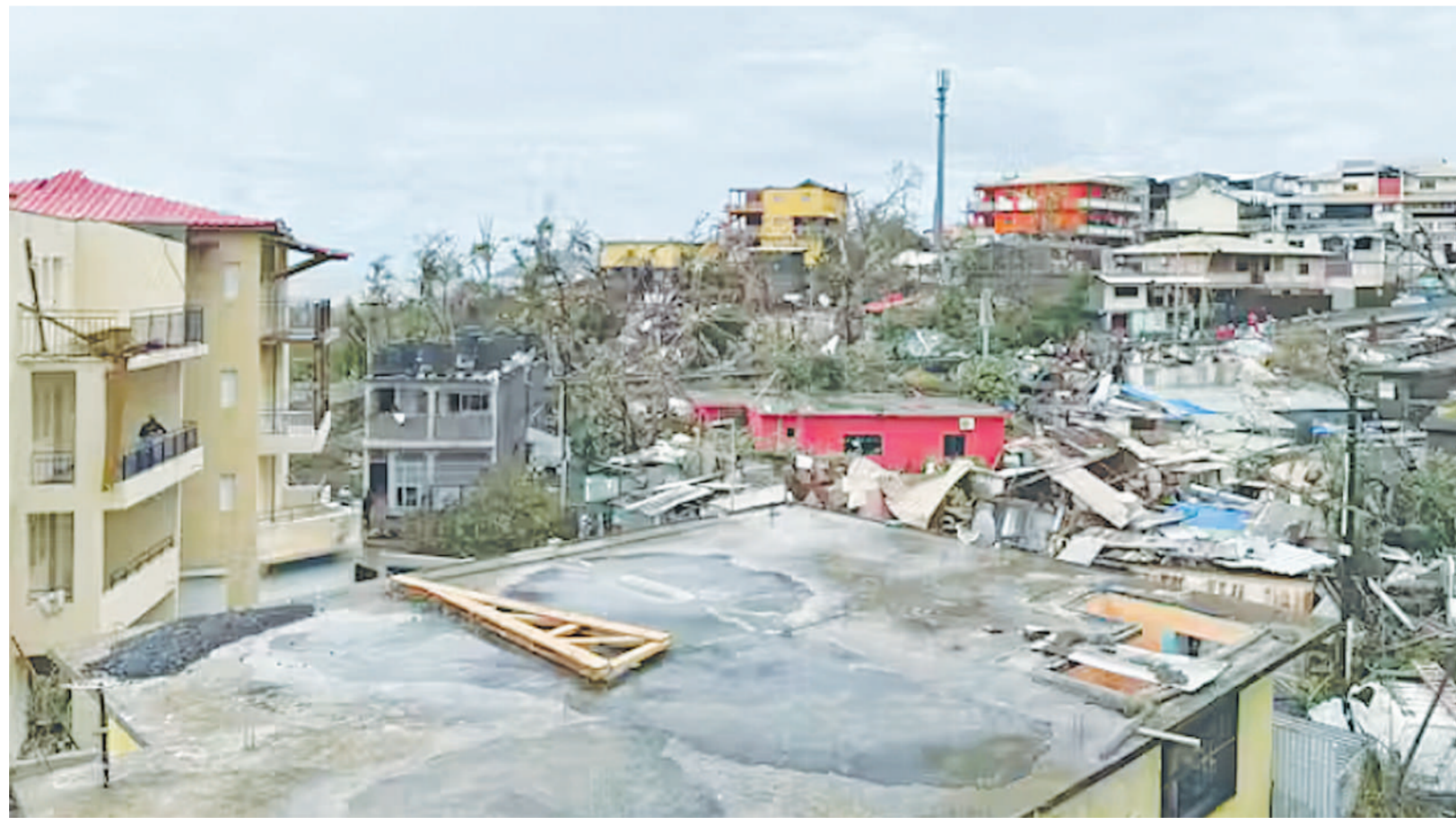
Damaged houses in Mamoudzou, in the French Indian Ocean territory of Mayotte on December 16 2024 after being battered by the islands' worst cyclone in nearly a century
