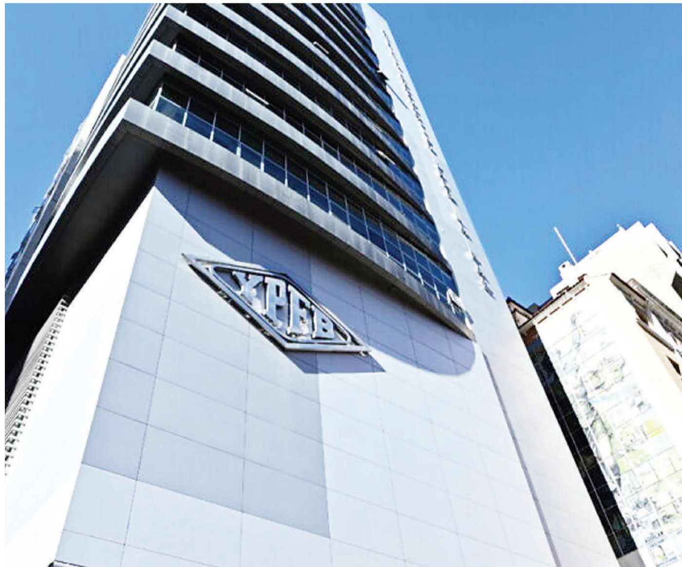
A photo of the 15-story building of the headquarters of Yacimientos Petrolíferos Fiscales Bolivianos (YPFB), located in La Paz, where the executive and organizational offices of the government-owned oil company have been operating since 2018. CREDIT: Franz Chavez/IPS
