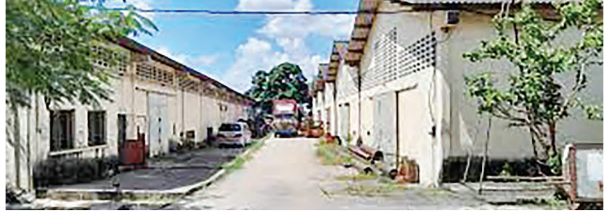
Current state of Urafiki Textile's warehouse facilities. File Photo
