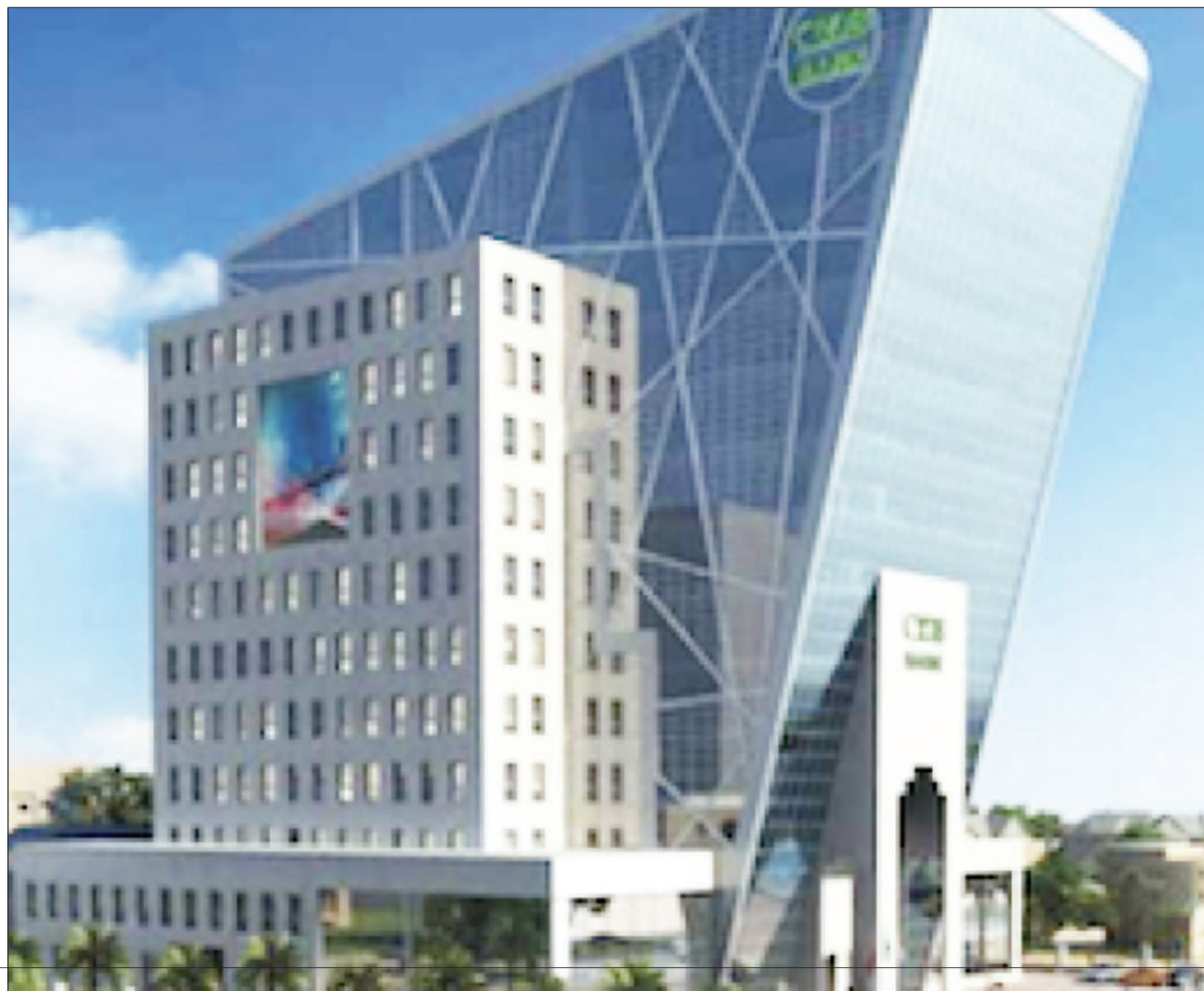
CRDB Bank Plc's new head offices in Dar es Salaam.
