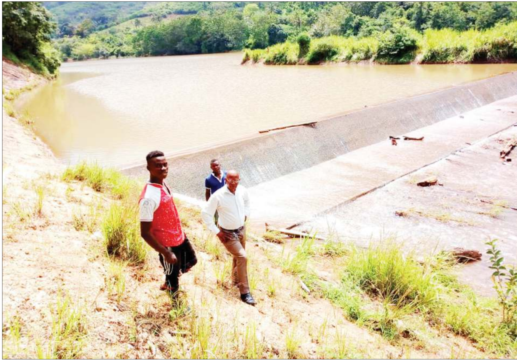
It must be shock and disbelief for these presumed residents of Misozwe in Muheza District, Tanga Region, at the weekend after they witnessed the havoc the recent heavy rains have wreaked on the village's irrigation scheme. Photo: Correspondent Steve William
