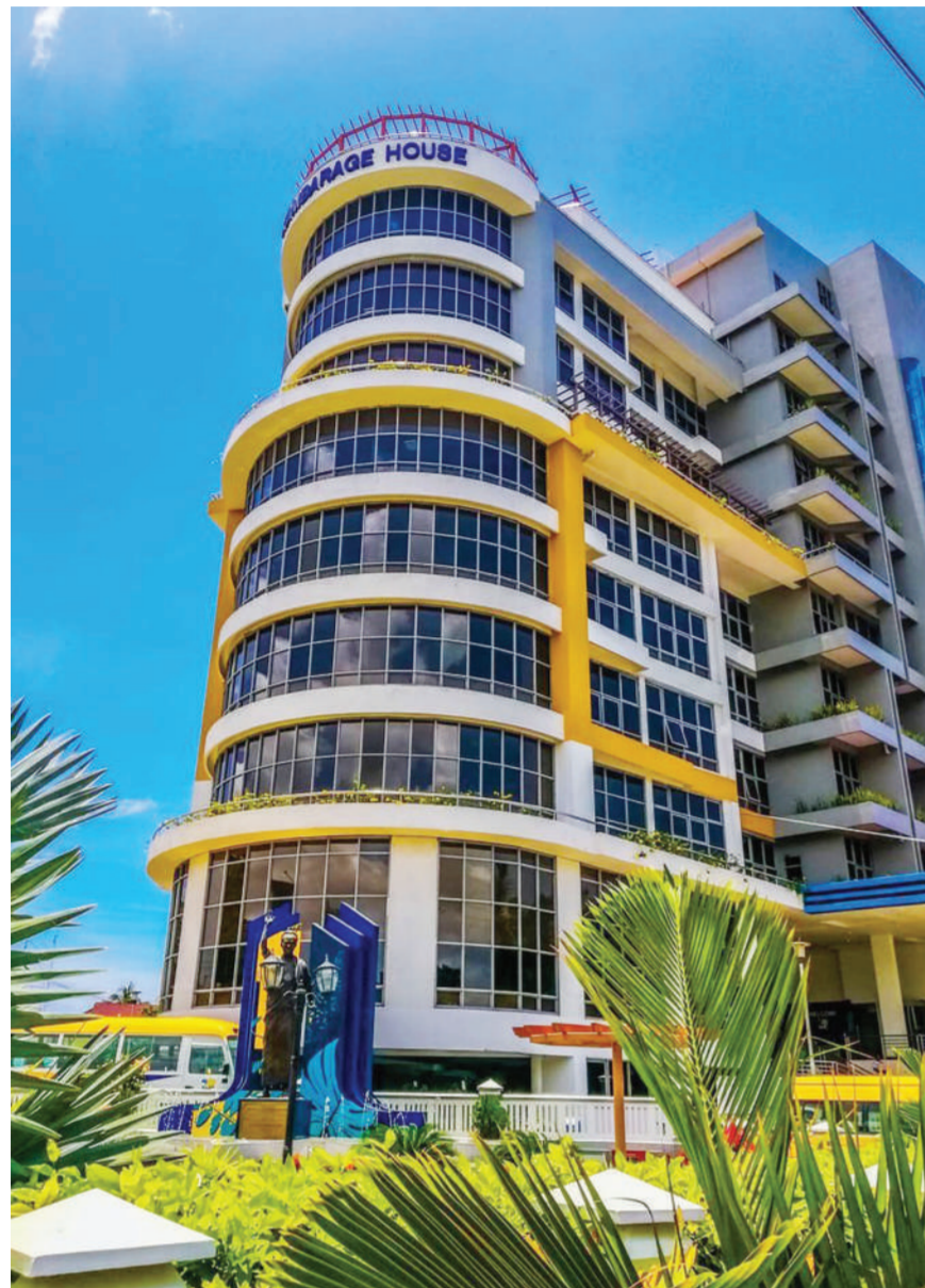
NHC headquarters in Dar es Salaam. The CAG has found serious weaknesses in the management of the partnered property investments. PHOTO/FILE
