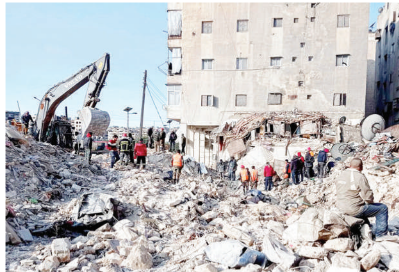
People search for survivors among the rubble of a building destroyed in a powerful earthquake in the al-Masharqa neighborhood of Aleppo city, northern Syria, on Feb. 6. Xinhua
