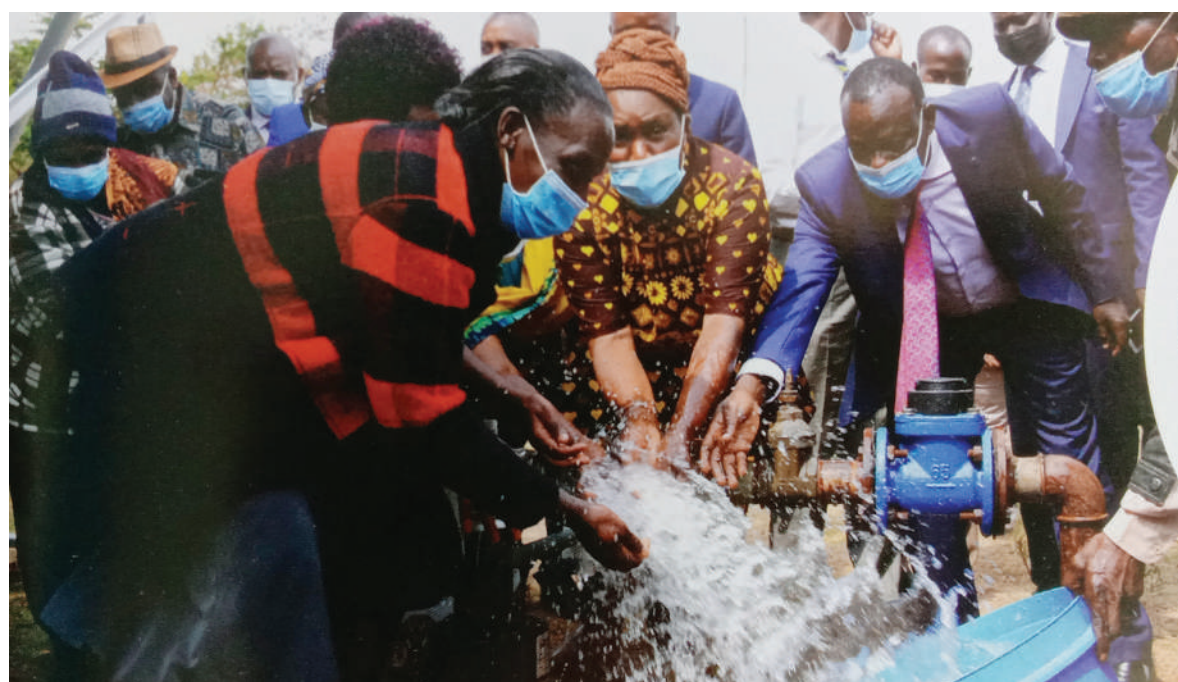
Tapping of underground water is very crucial for human development
