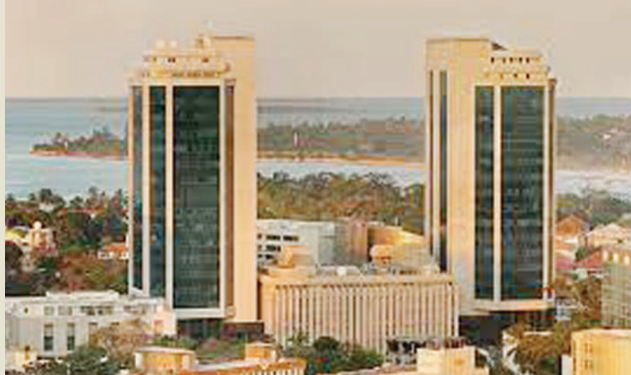
Bank of Tanzania headquarters in Dar es Salaam
