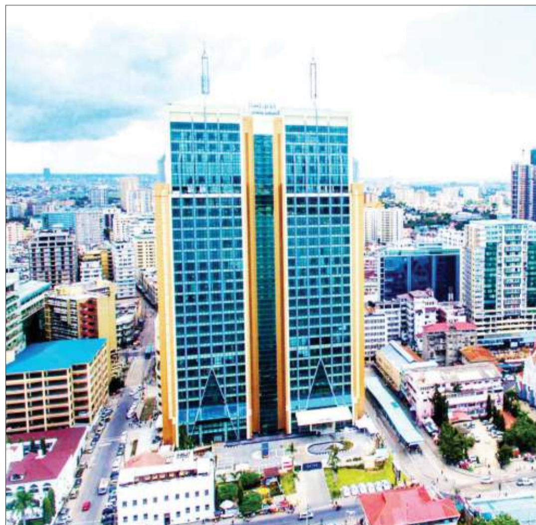
View of New Mwalimu Nyerere Foundation Square building located in Dar es Salaam after completion. The 30 story building built by the Chinese Construction company CRJE (East Africa) Ltd is expected to be launched soon. Photo: Guardian Correspondent
