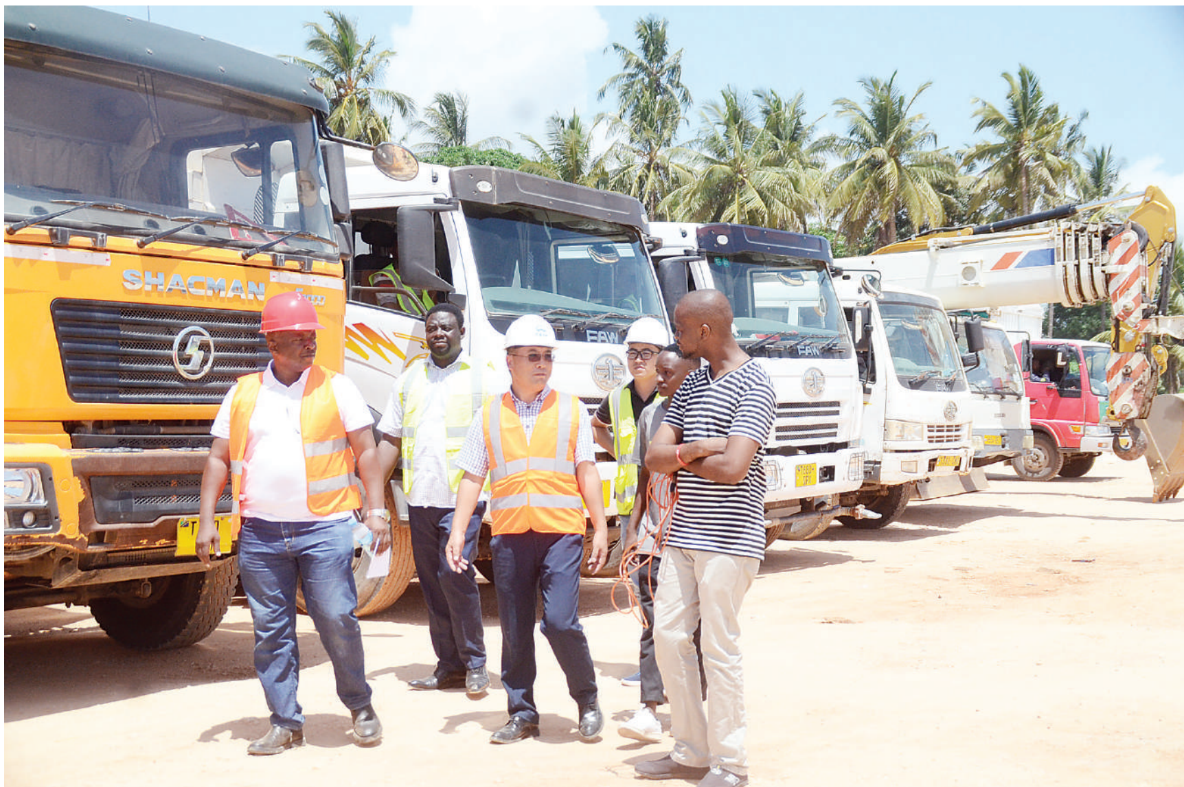
China Railway Construction Engineering Group's director of projects, David Zhou (C), briefs journalists in Dar es Salaam yesterday on the resumption of the construction of the 1.2-km road section between Nyerere Bridge and Ferry-Kibada in compliance with President John Magufuli's recent directive to that effect. Photo: Guardian Correspondent
