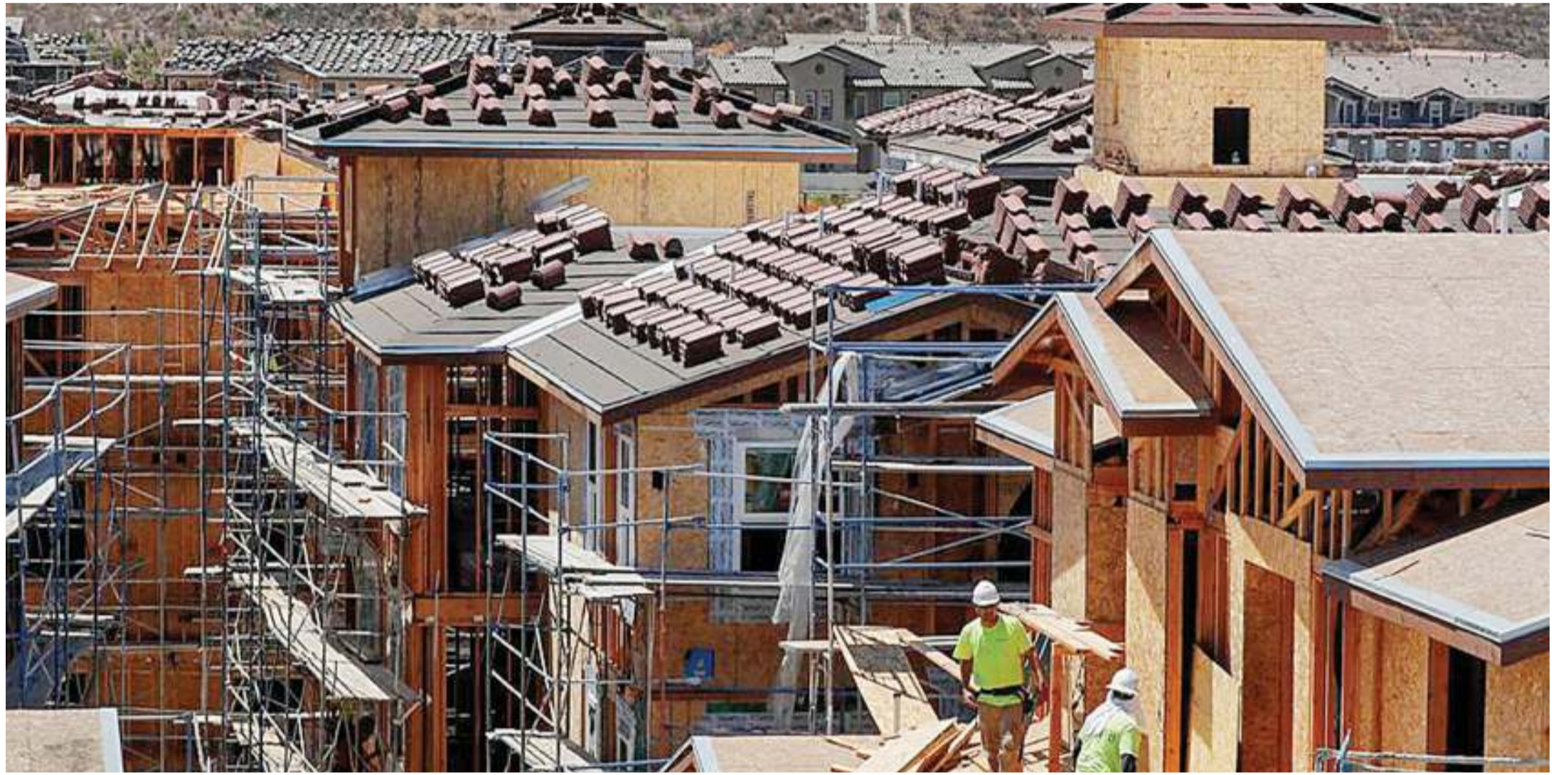
Construction of wood-frame houses going on in Durham, North Carolina.
