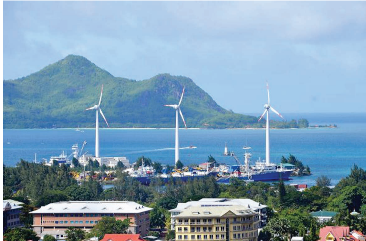
A wind farm in Port Victoria on the main island of Mahe in the Seychelles is contributing to the renewable energy transition of the small island state located east of the African continent. Credit: Commonwealth Secretariat
