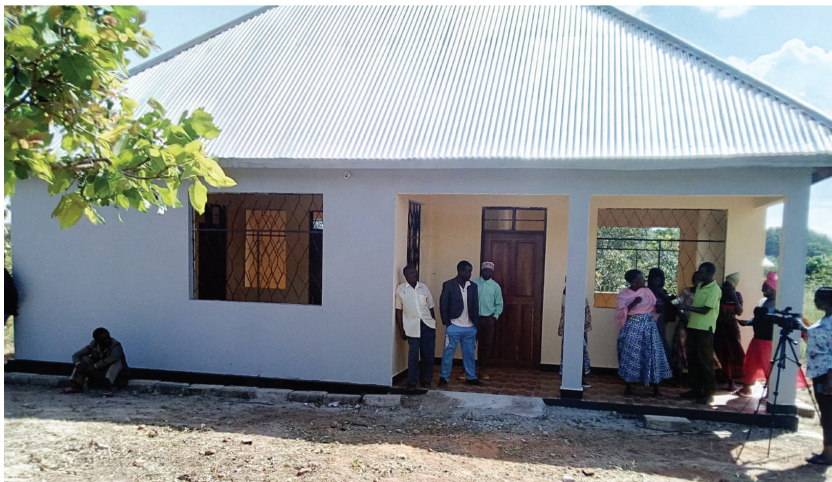
A maternity ward building in Kitanda village put-up with funding from the forest conservation project.
