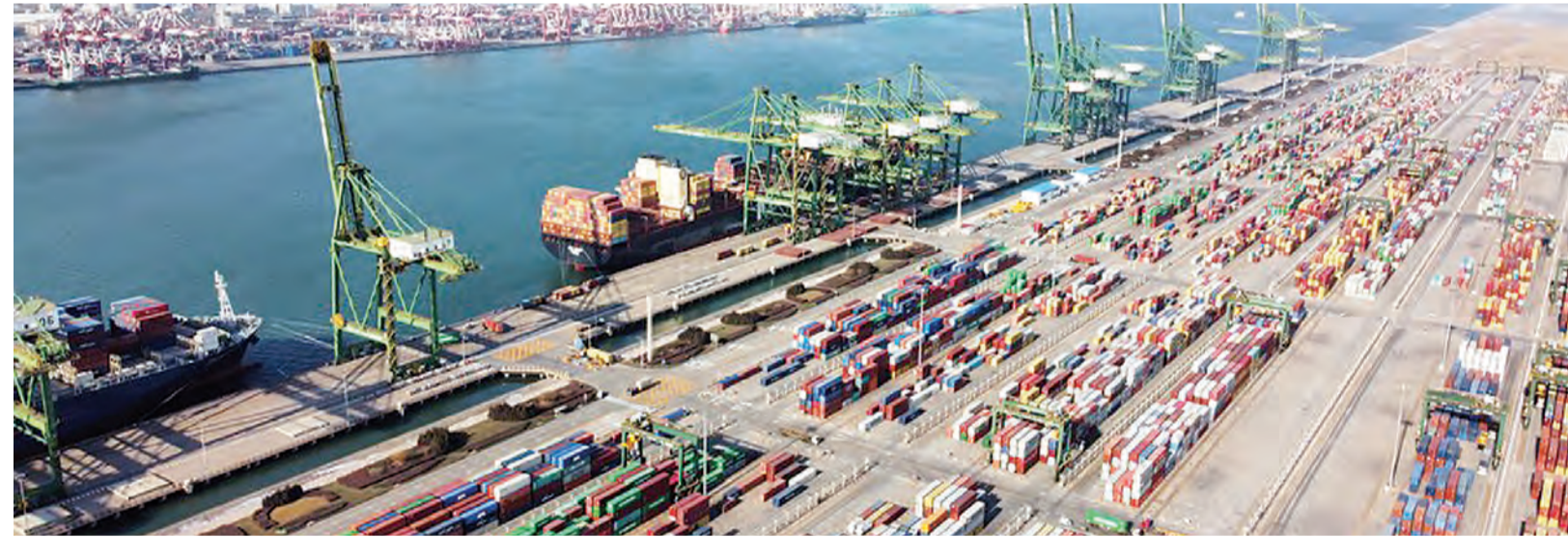
Aerial photo taken on Jan. 11, 2021 shows a view of the Pacific international container terminal at Tianjin Port in north China's Tianjin Municipality. (Xinhua)
