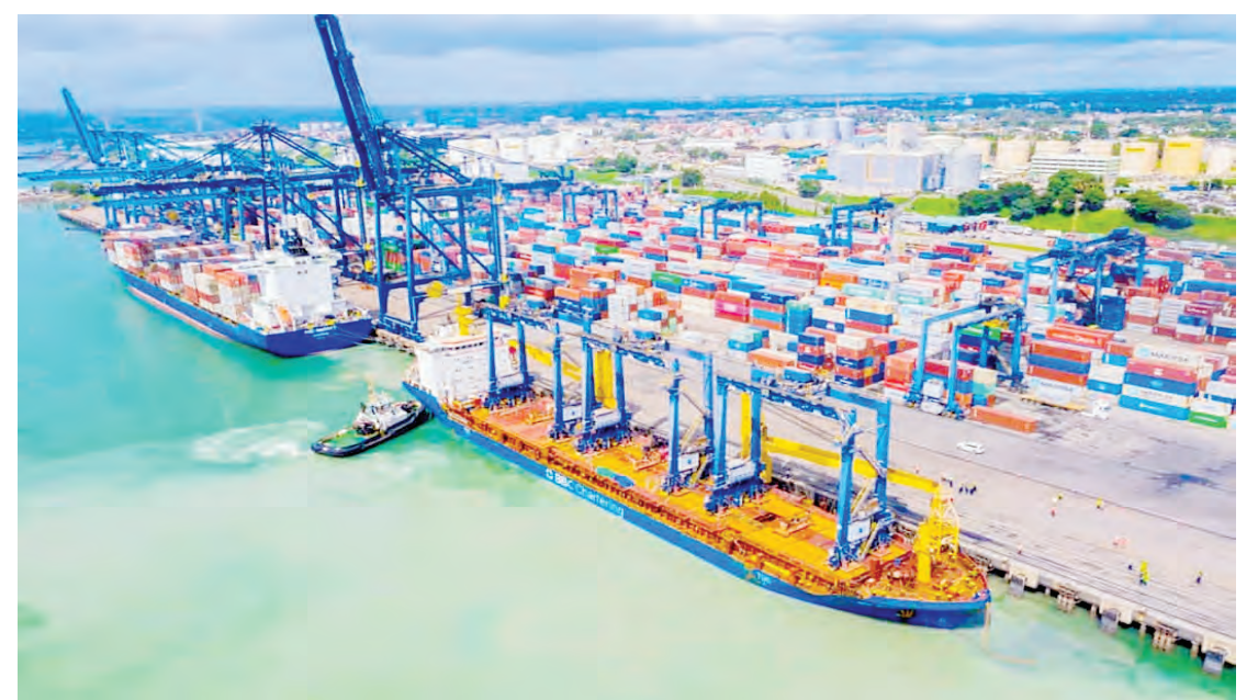
TICTS' ongoing investment program saw the arrival of three additional rubber-tyred gantry cranes earlier this year.
