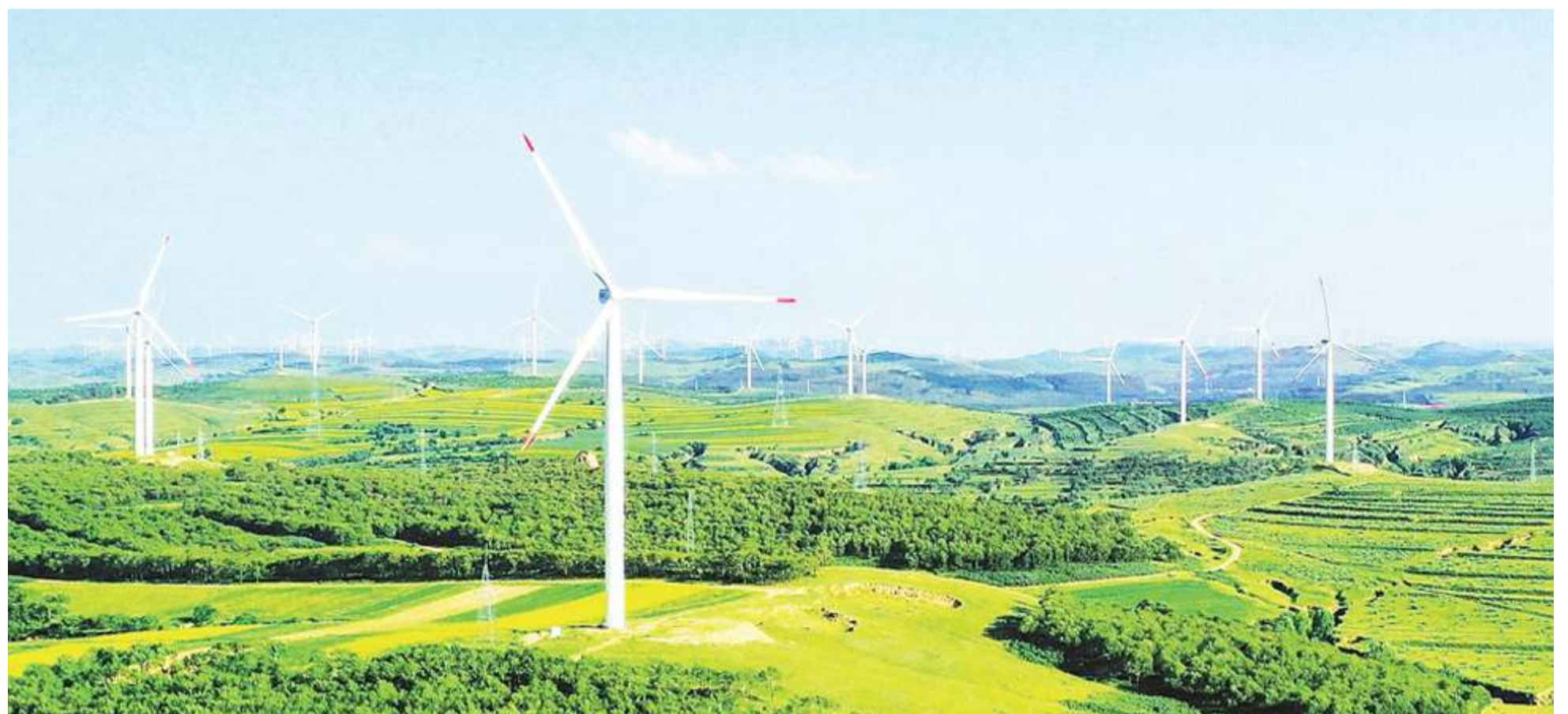
Wind farm of Jinneng Group in North China's Shanxi province.
