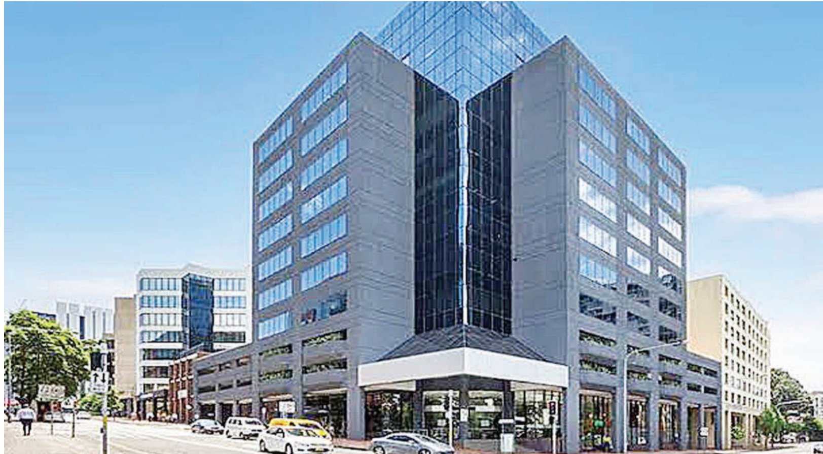
SC Capital's Two Wentworth Street building.
